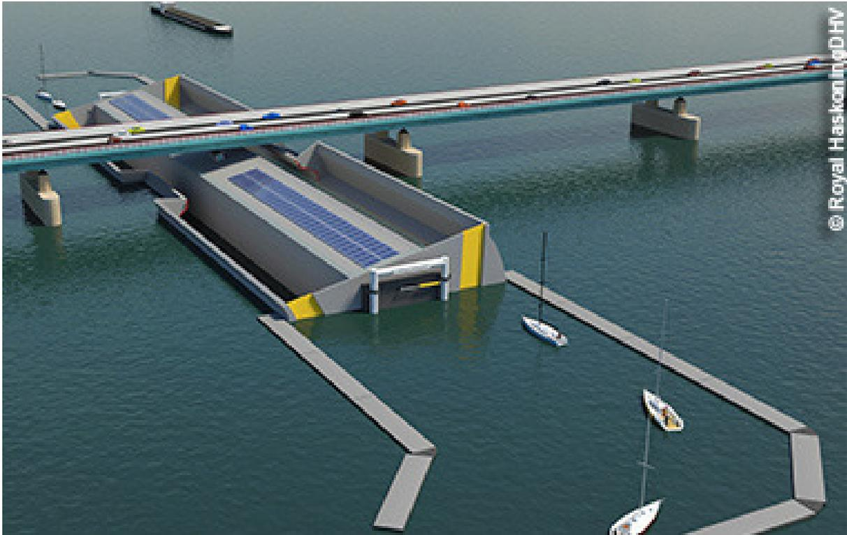
***As boats enter the lock, it is tilted up approximately 16 degrees. Once the boats are inside and the watertight doors are closed, the lock tilts down 32 degrees, adding 8 m of clearance. © Royal HaskoningDHV***
