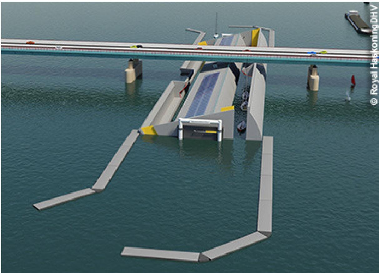
**Solar photovoltaic panels provide power to tilt the lock, which moves slowly and displaces no water. © Royal HaskoningDHV.**
